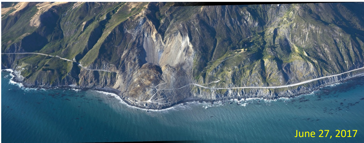
Figure 2. Oblique aerial photographs (stitched together by UCSC using SpinPanorama) of the Mud Creek Landslide taken June 27, 2017 and provided by Jonathan Warrick (U.S. Geological Survey).
